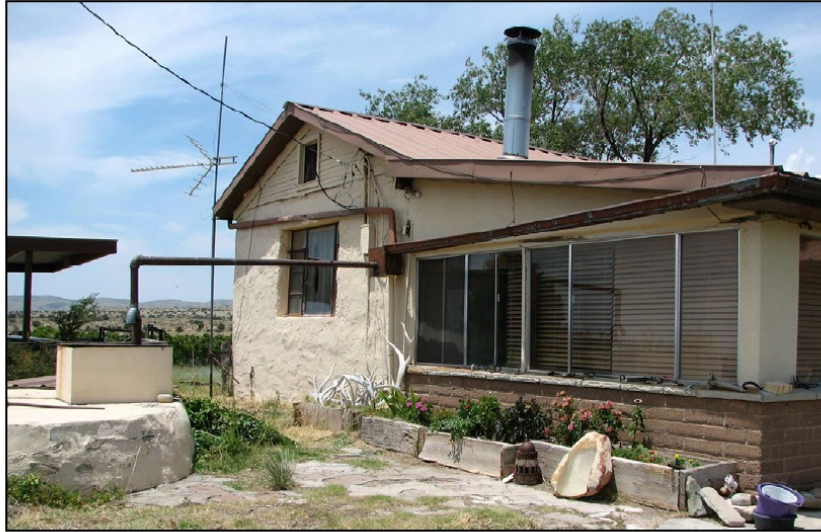
Fig. 10-20. A system for collection of water off the roof of a residence on the Black Hills Ranch, formerly the Nalda Ranch, east-northeast of the Trinity Site. The cistern to the left, which was damaged by the Trinity blast then repaired, is still in use today.
